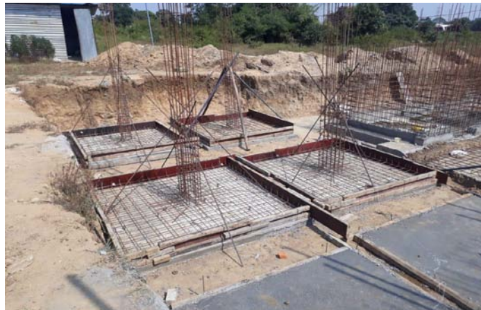
Fig. 2 Construction Sites in Central India Region
